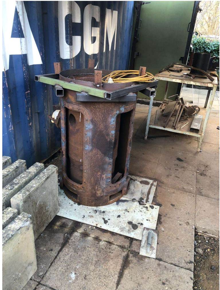
The coke fired boiler from the sleeping car with the crane lifting attachment still attached (Above).
