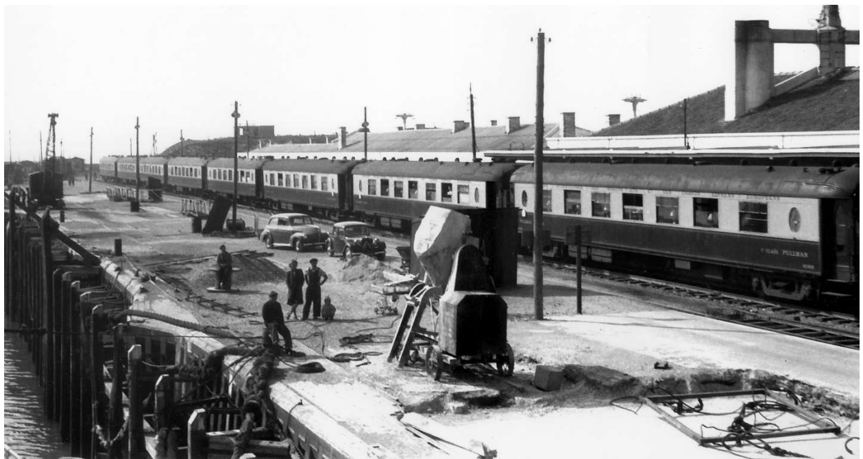
An immediate post-war shot still with visible war damage in repair in Calais-Maritime. We see a total of 8 Pullman cars of the type Côte Azur standing in a long row, these were travelling in the Flèche d'Or to Paris. In front as the first one the WSP 4149, the numbers of the other coaches are not recognisable. Not only 4149 is missing the monogram, but also some of the cars further back, only the second car has a recognisable monogram. This was probably a victim of war production as important raw materials under German forced administration. Photo: Mike Morant, https://mikemorant.smugmug.com/ , coll. Dirk Frielingsdorf
