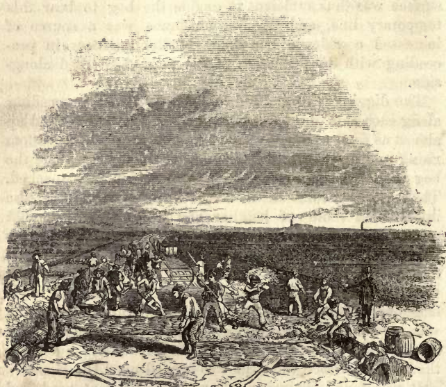
Chat Moss. Works in progress.
