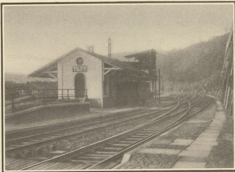
TILFF — HANGAR AUX MARCHANDISES
